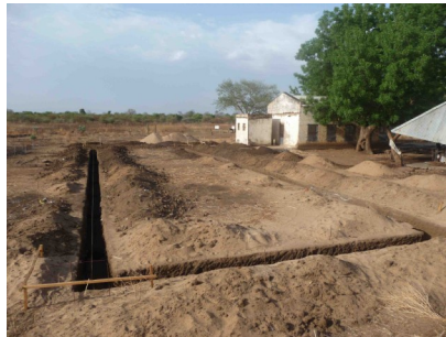
Above: First, the foundation is laid.
